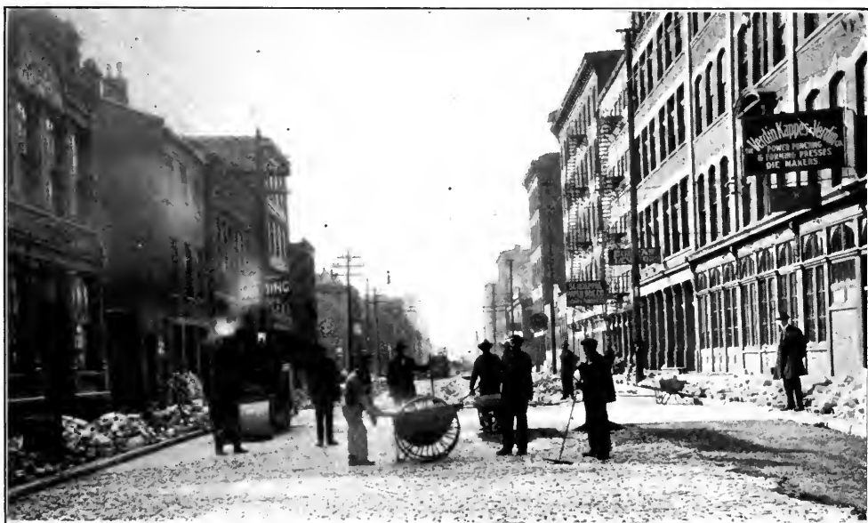
APPLYING A FLUSH COAT TO GRANITE BLOCK PAVEMENT ON SECOND STREET, CINCINNATI, OHIO
